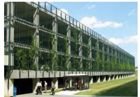
Census Bureau, MD. Green Facade trellis system shortly after installation. (2006)
