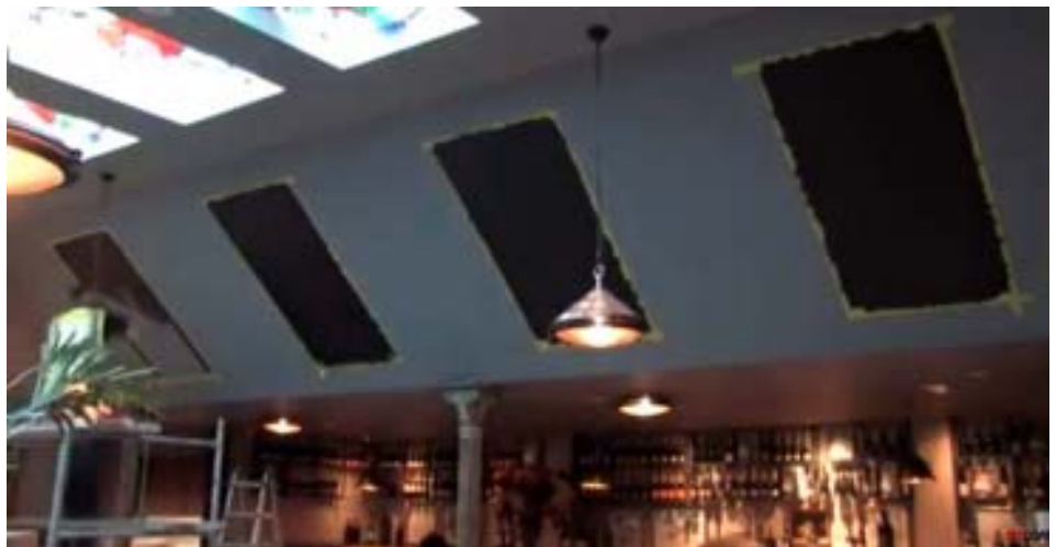
IR Paint on Restaurant Ceiling, before finish paint is applied.
