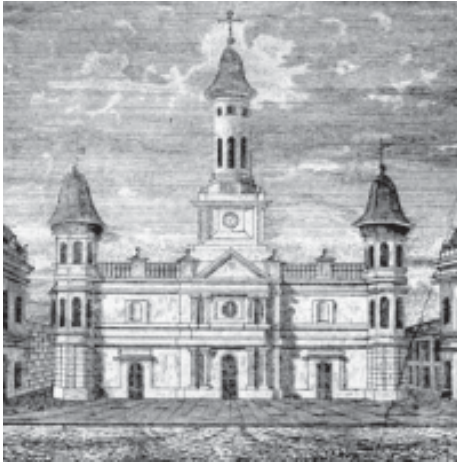
St. Louis Cathedral, 1838, with Latrobe's central tower design.
