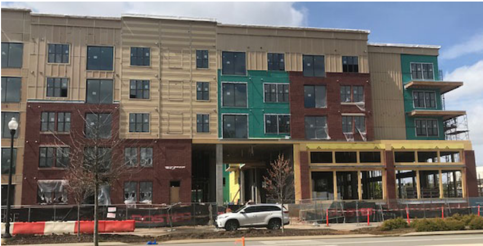
This 5-Over-1 under construction illustrates the concrete to wood transition, and the design, even unfinished, clearly indicates the different usage types intended.
