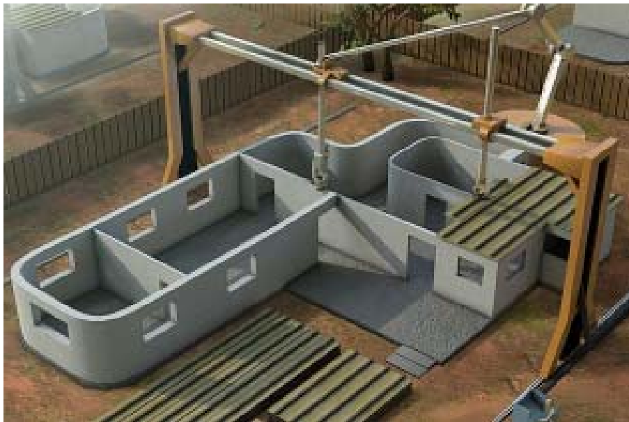
3d Concrete Printer by Scott Lewis
